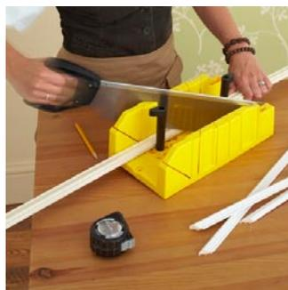
To make a corner, cut the molding at a 45-degree angle using a miter box.
